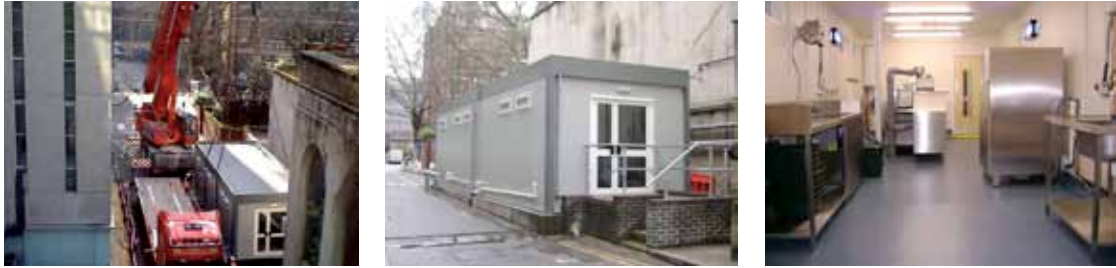
The multi award-winning CompPod at Imperial College occupies a small footprint yet processes in excess of 2 tonnes of food waste every week.
